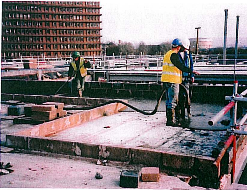
Figure 2: Placing the foam concrete on the roof.
