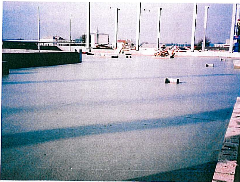
Figure 4: The finished foam concrete roof slope.
