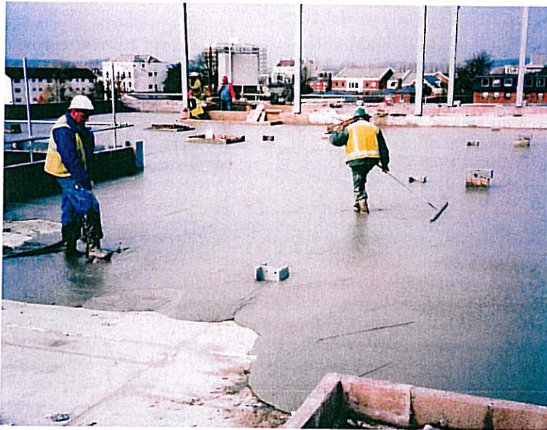
Figure 3: Float-finishing the foam concrete.
